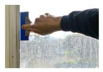
After trimming, mist the entire surface of the film, squeegee it again in the same pattern as directed in Step 7. This time bump the frame. Press firmly to remove all the water that you can. Start at the top of the window, squeegee from the center to the left, then from the center to the right. Repeat this process until you reach the bottom of the window. At the bottom squeegee down across the window from a few inches above the frame and bump the frame all the way across the bottom.
